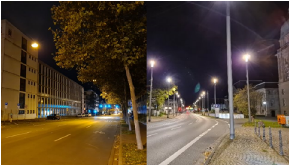
Figure 4: The urban traffic area offers great potential for increasing efficiency due to existing street lighting
