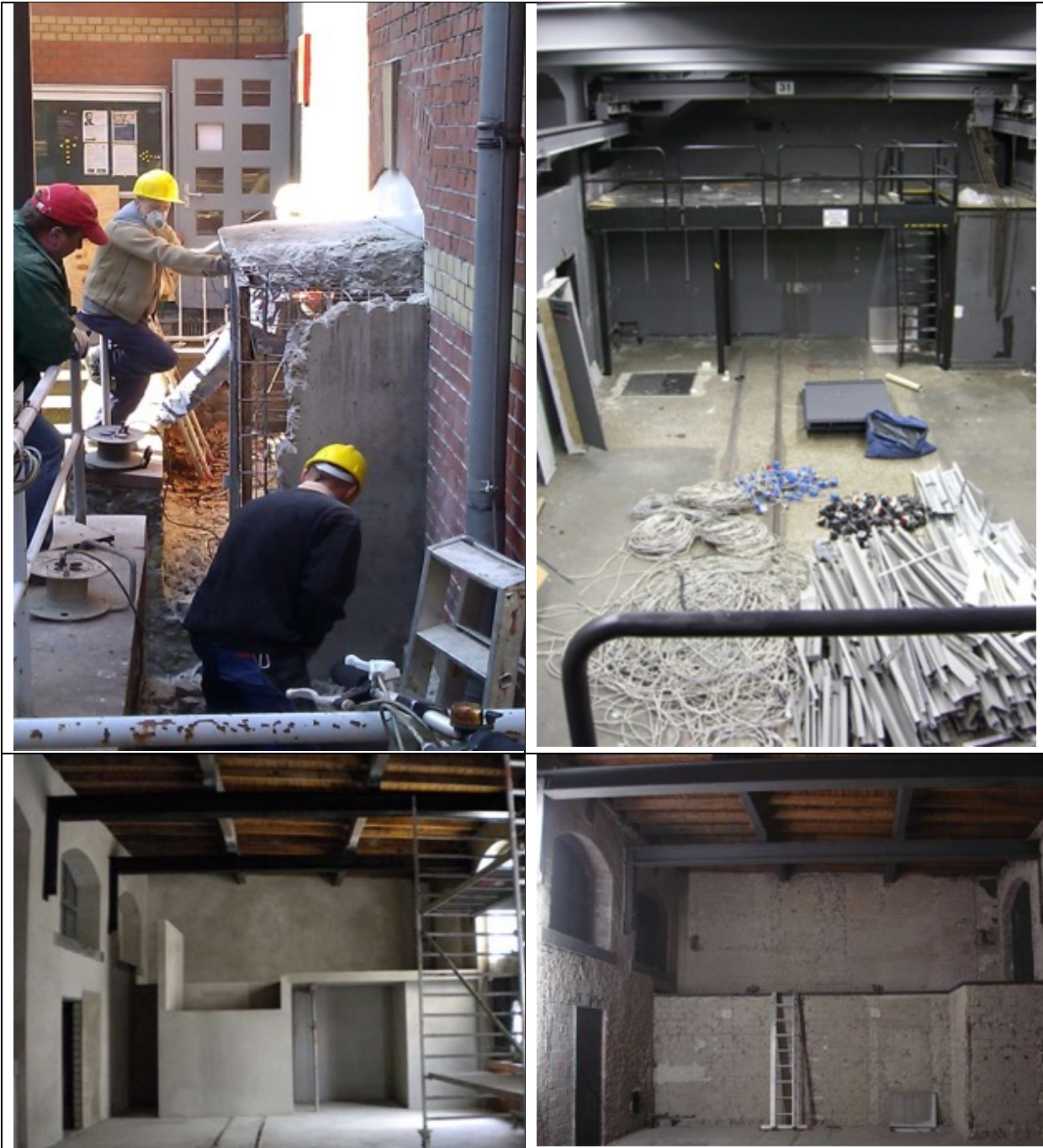
During Renovation Outside and Inside Building 17
